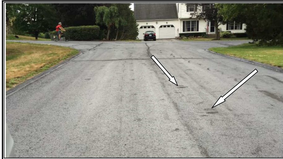
Photo #2: Tire tracking from bituminous crack filler
