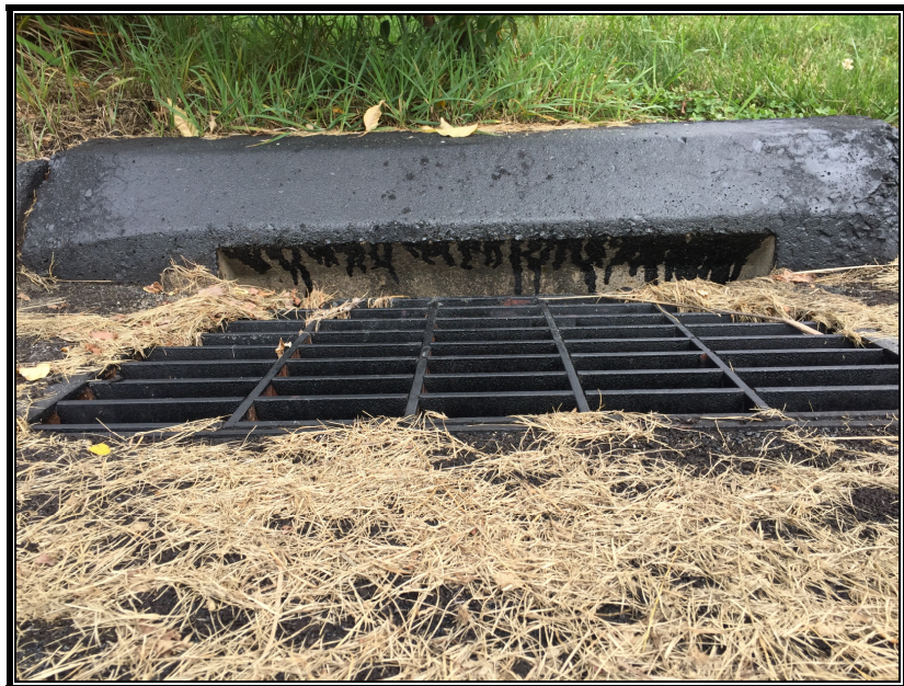
Photo #5 PDC overspray into catch basin throat
