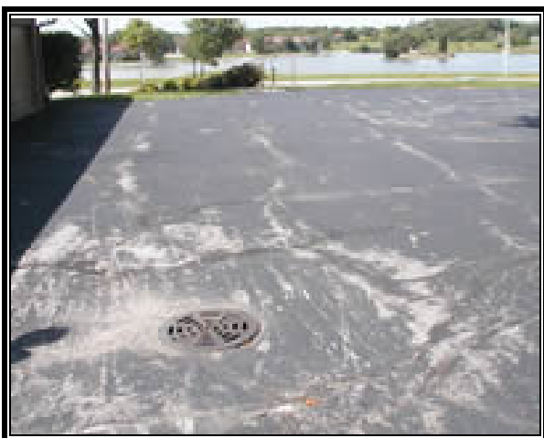
Photo #6: Worn sealcoat surface – note proximity to storm drain.
