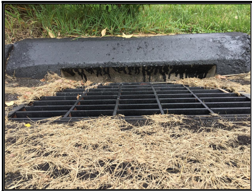
Photo #5 PDC overspray into catch basin throat
