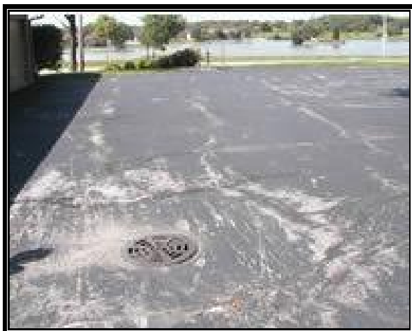
Photo #6: Worn sealcoat surface ó note proximity to storm drain.
