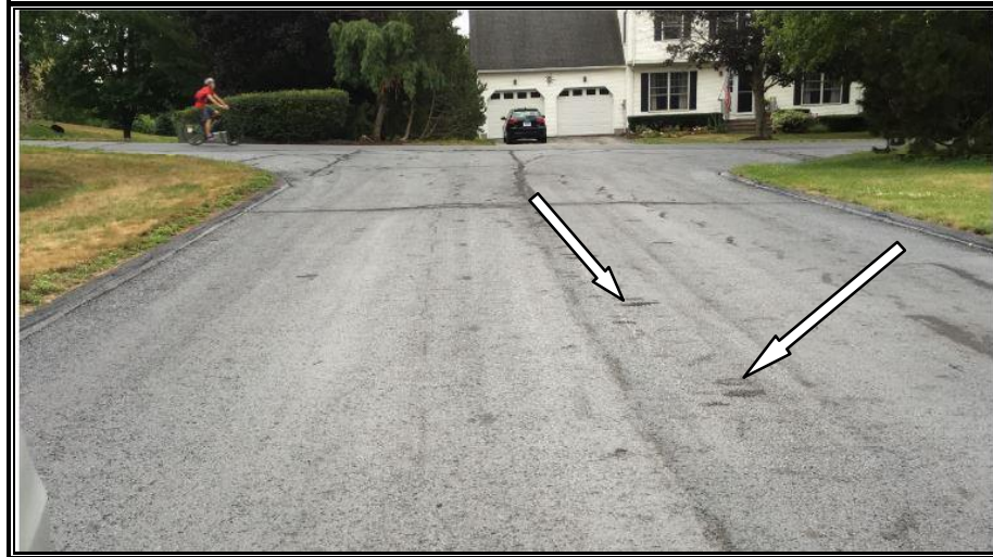
Photo #2: Tire tracking from bituminous crack filler
