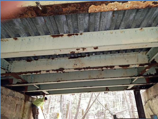
Typical Underside of Superstructure Prior to Repairs Completed 2021
