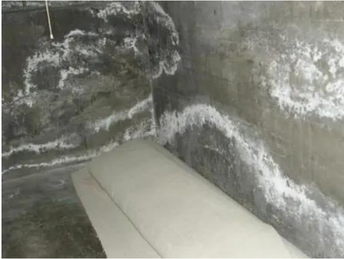
Efflorescence
