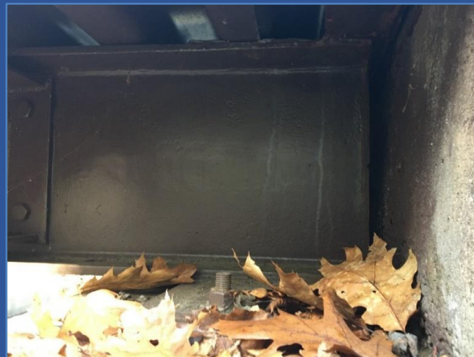
Beam End Repair Completed 2021
