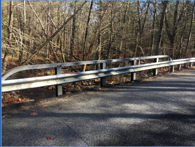
Eastern Bridge Rail – Does not Meet Safety Standards
