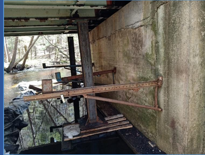
North Abutment with Exposed Scour Wall (Site Visit Spring 2021)
