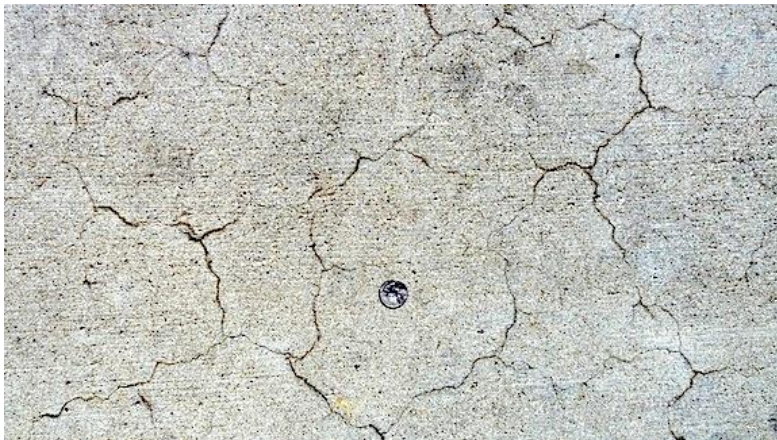
Map Cracking
