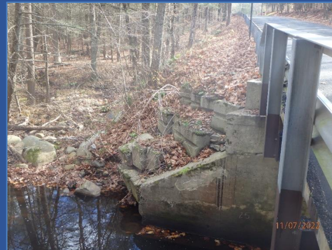
Southeast Wingwall. Note concrete blocks at embankment slope (typical at all wingwalls).
