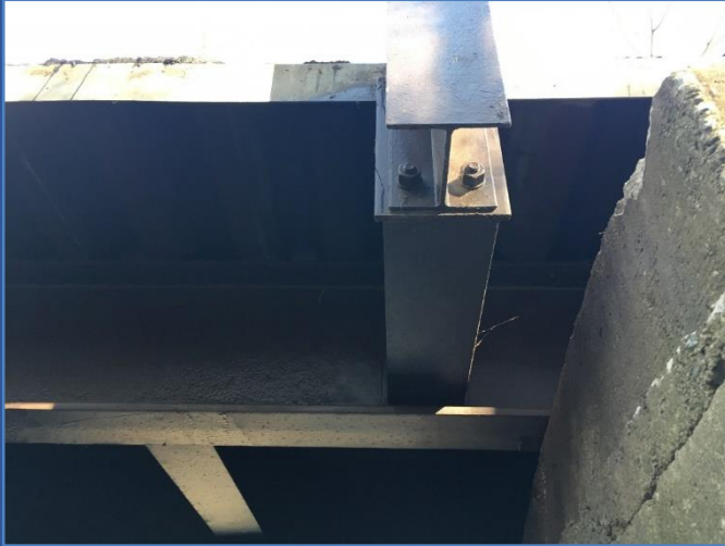
Repaired Connection of Bridge Rail Post to the Fascia Girder Completed 2021
