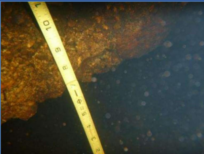
Undermining at South Abutment Scour Wall (Inspection Report, January 25, 2022).
